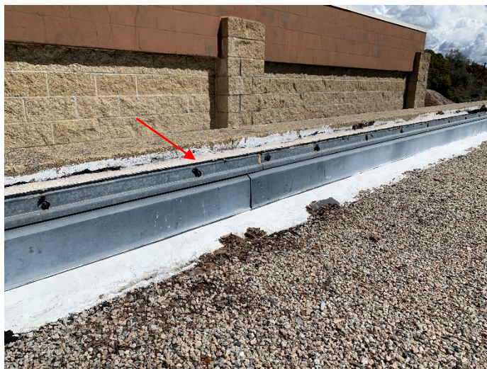
Photo #4: Drama classroom roof, view of east parapet wall, showing asbestos-containing off-white flashing caulk
