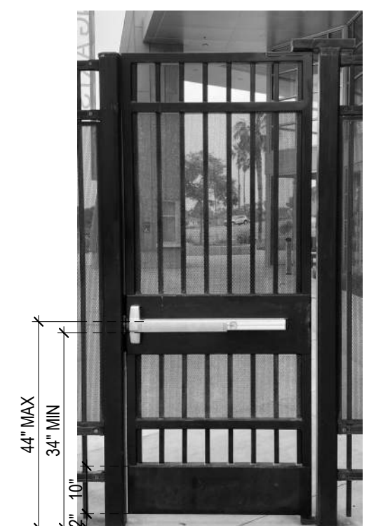
INTERIOR PUSH SIDE
